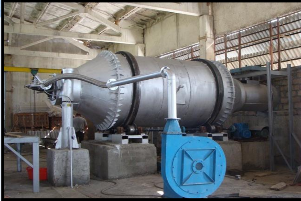
Battery Plate Making Workshop
